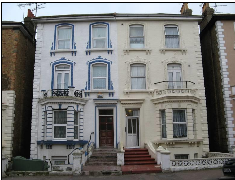
These properties in Athelstan Road would benefit from grant aid to restore lost architectural features
