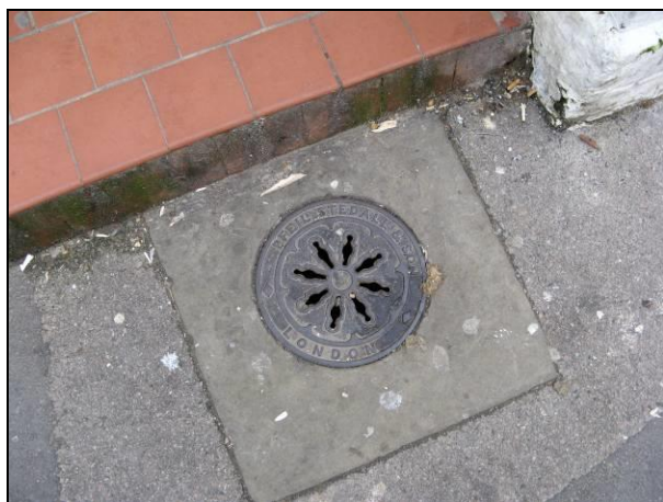
A cast iron coal hole cover in Athelstan Road
