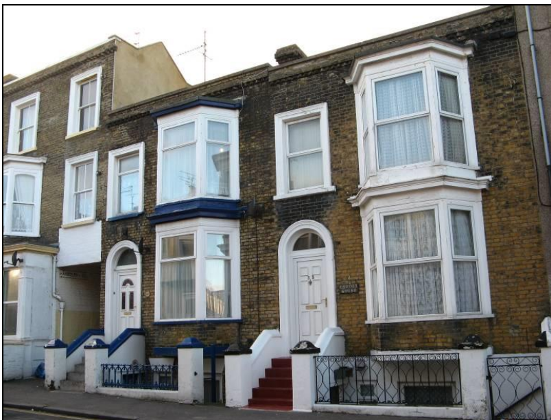
Protect the boundaries to these historic buildings in Ethelbert Road
