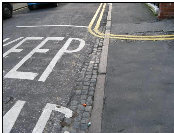
Granite setts and kerb detail, Ethelbert Road
