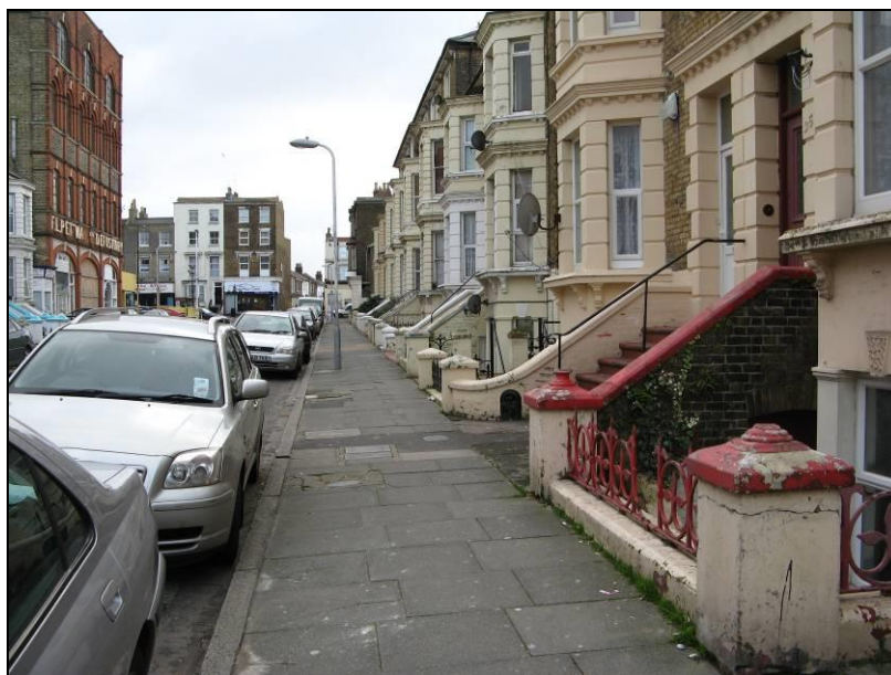
Improvements are needed to the pavements and street lights in the Conservation Area
